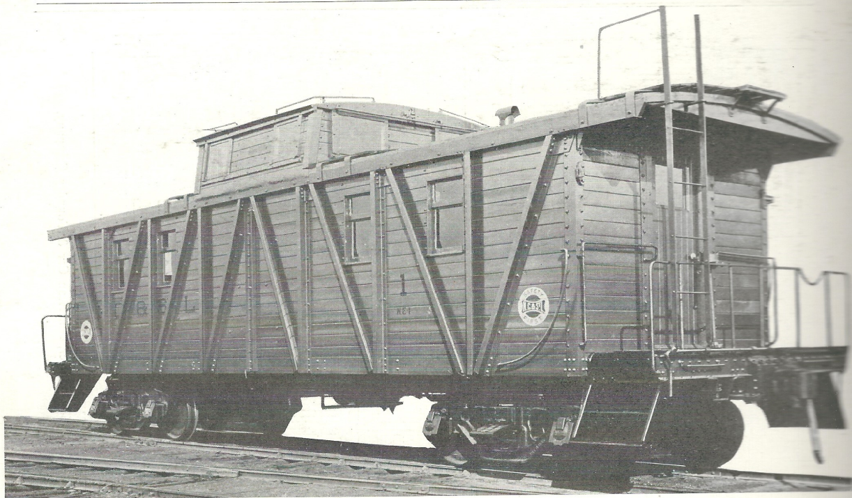
Fig. 261—Steel Frame Single Sheathed Caboose. With Specially Constructed Underframe for Use in Heavy Pusher Service. Nashville, Chattanooga & St. Louis Railway. (See Figs. 262-266.)
