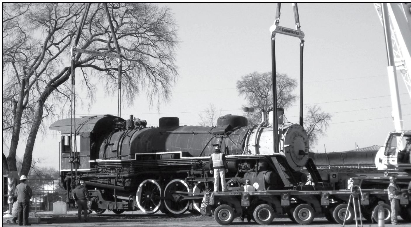
The 350,000-pound Locomotive Was Lifted with a 200-ton Capacity Crane and a 400-ton Capacity Crane, the only 400-Ton Crane in Alabama.
