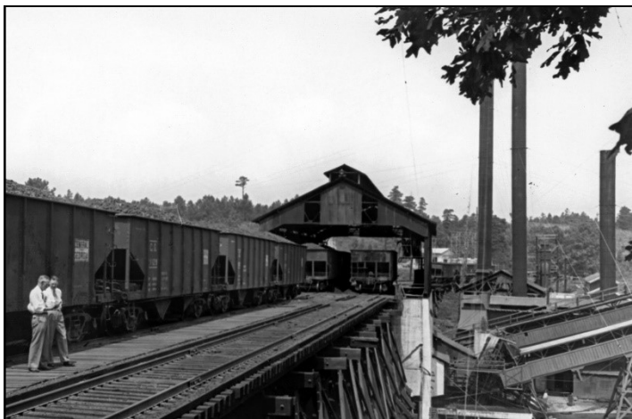
View from the dump track at the Colgate washer plant showing cars on the dump and cars waiting to roll into the dump. (Clemons, CoG photo).
