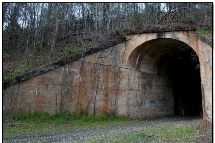
Margaret Branch tunnel under the SAL mainline (Clemons)
