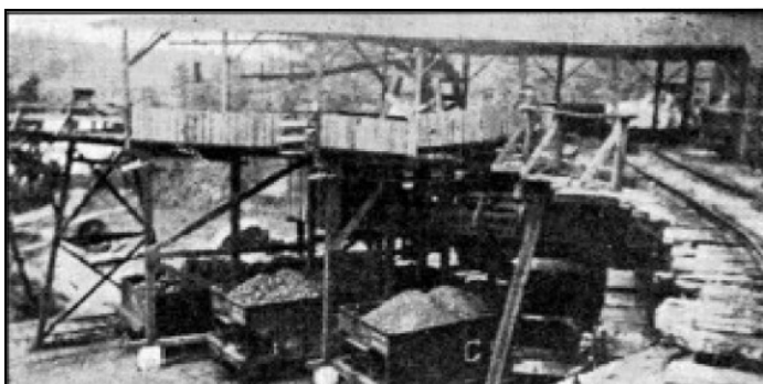
Loaded cars at tippel, likely Margaret No 3 c 1921 (Clemons, CoG Magazine). Coal was sorted by size at the tippel with shaker screens, larger sizes being picked at the tippel, ready to ship, and smaller sizes sent to the washer.
