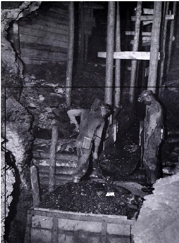
Miners working the "Big Seam." Note the chute between the men bringing coal down from the working face. The Big Seam (Mammoth) was about 11 feet thick with a top and bottom "bench" separated by a layer of rock. Different methods were used as shown in the section view in the right image. This appears to be the method in the top diagram. In the diagram below, we see this in plan view. Note the typical slope (pitch) of 20 degrees. (Denny Explosives Engineer Magazine, 1944.)
