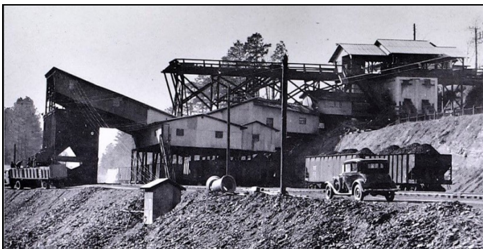
Acmar No 8 tipple, likely the last tipple to be built. The head house and dump on the right, screening house in the middle, with loadout to rail cars below and the truck dump on the left. Truck sales continued to grow during the 1940's. (Denney, Explosives Engineer, 1944)
