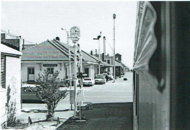
The former ACL depot at Valdosta was built to the standard tile roof and brick construction commonly found on larger station buildings in Coast Line territory. All the markings of a small-town depot are present—the ubiquitous train order semaphores, a green Railway Express Agency truck picking up express, even a couple of the local citizenry propped up in a window sill taking shade from the morning sun. The block signal in the foreground is the approach to Southern's GS&F crossing just to the west of the station. —Marvin Clemons photo
