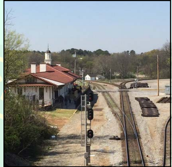
View of joint L&N/Southern Decatur depot looking south. L&N track to Birmingham curves left, Southern to Memphis curves right. (Clemons collection)
