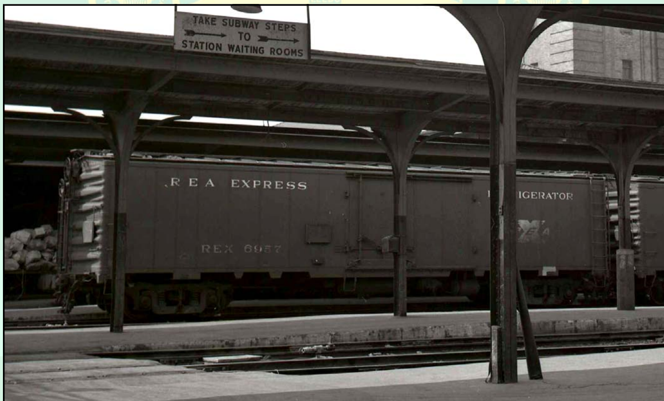
In October 1968, a REA Express car containing refrigerated produce awaits its connecting train at Birmingham Terminal Station. (Don Phillips photo, Marvin Clemons collection)
