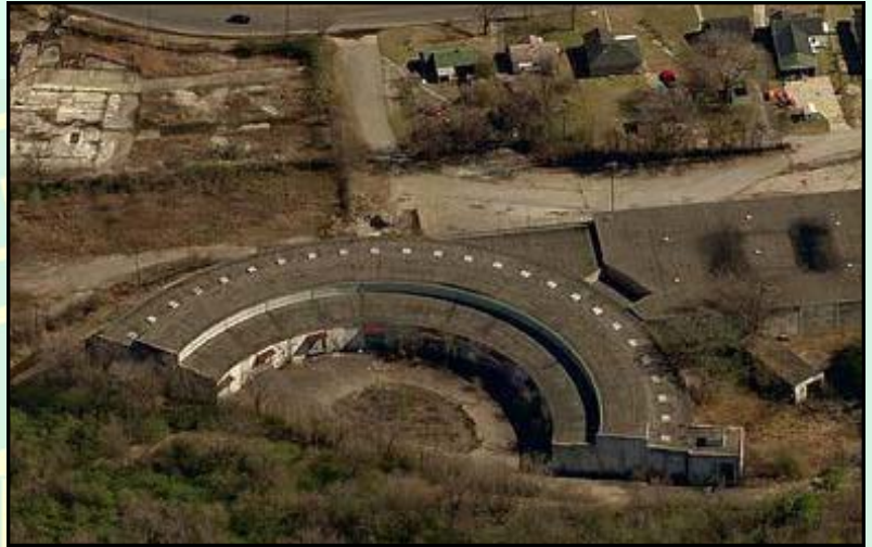
Remains of Southern Railway's Finley roundhouse
