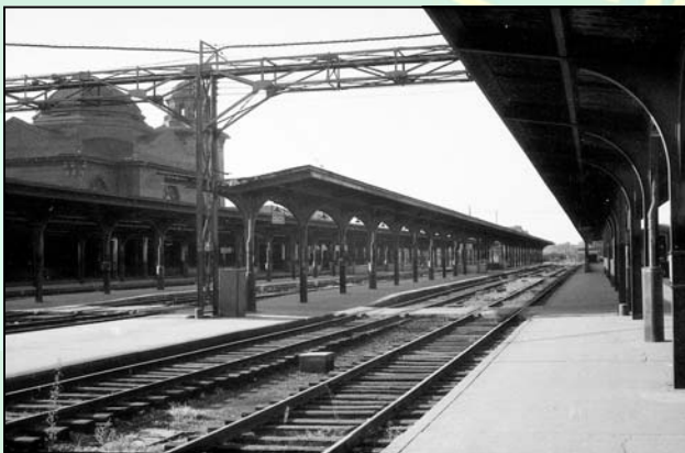
A vacant and forlorn Terminal Station in 1969
