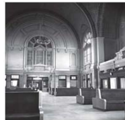
Main Waiting Room, Southwest View
