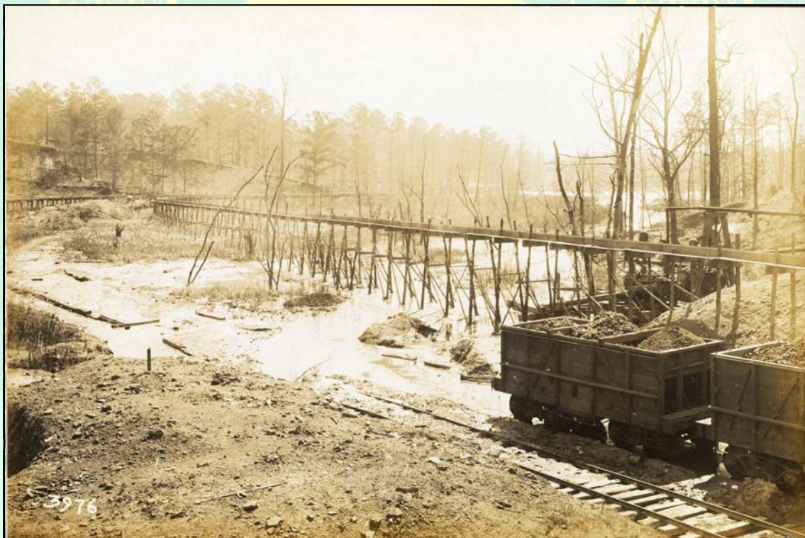
A view of the settling ponds from one of the washer sites showing sluice boxes carrying water. The ponds created system of ponds with water flowing from one to another before eventually leaving the property. These required the construction of levees which had to be maintained and might break causing downstream damage. (U of A, Hoole collection)
