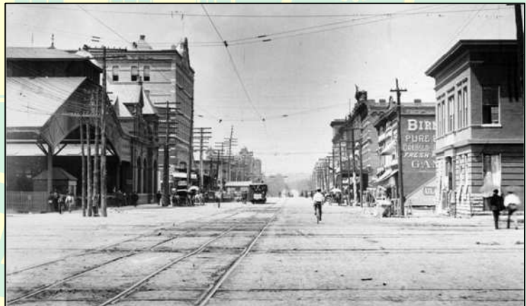
This early view is looking north along 20th Street with two streetcar tracks passing the L&N Station at left. Birmingham Public Library
