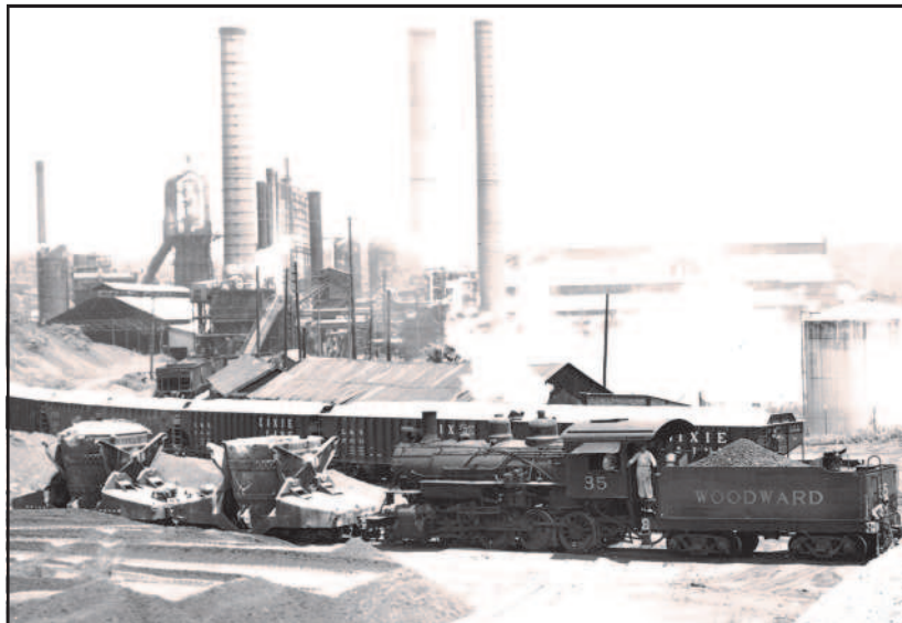
Woodward "Mike" at work — Woodward Iron Co. 2-8-0 #35 (Baldwin 1922) has hot metal ladle cars in tow as it backs up the hill from behind the blast furnaces. This photo was taken in May 1959 during a brief revival of steam locomotive use at Woodward. (Photo by Thomas Lawson Jr.)
