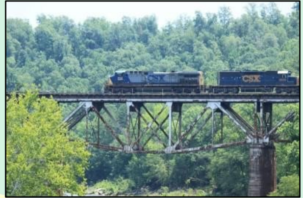
Mulberry Fork Bridge
