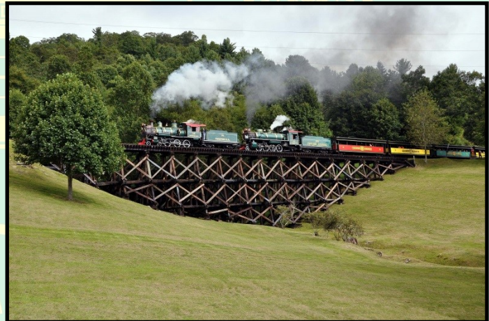
Sunday morning doubleheader charging across the trestle
