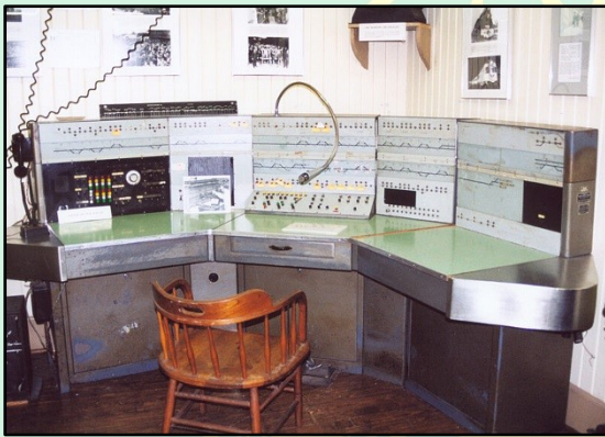
Birmingham Division CTC control panel
