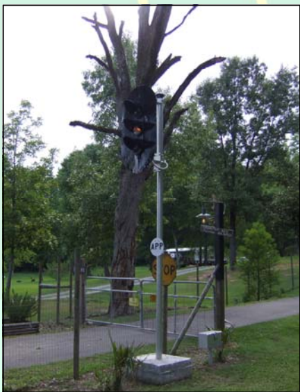
An approach signal protects the driveway
