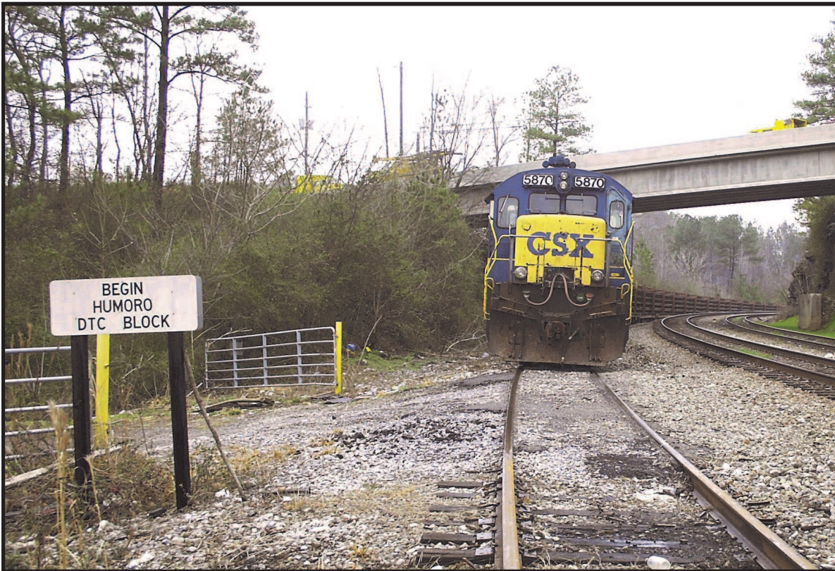
The rail removal is complete. More than seven miles of the Cane Creek branch has been loaded on the rail train as it sits on the remaining rail of this historic branch, at a place once called Humoro. Humoro was a train order station when the Mary Lee Railroad interchanged with the Cane Creek branch. The station was named in honor of Hugh Morrow, the President of Sloss-Sheffield Steel & Iron Company, and later, U.S. Pipe & Foundry.
